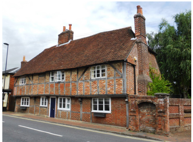
Figure 33 - No.8 Winchester Street
