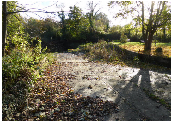
Figure 44 - Old slipway into river
