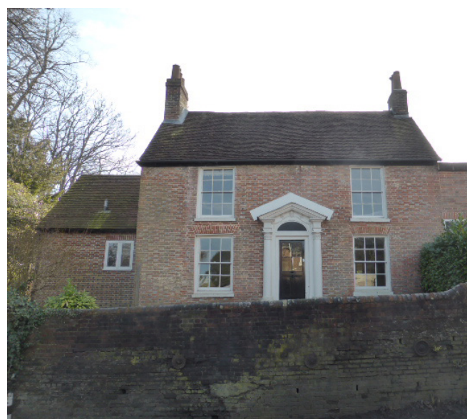
Figure 32 - No.16 Mill Hill
