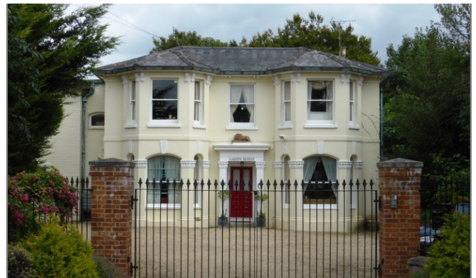
Figure 24 - No. 6 Winchester Street
