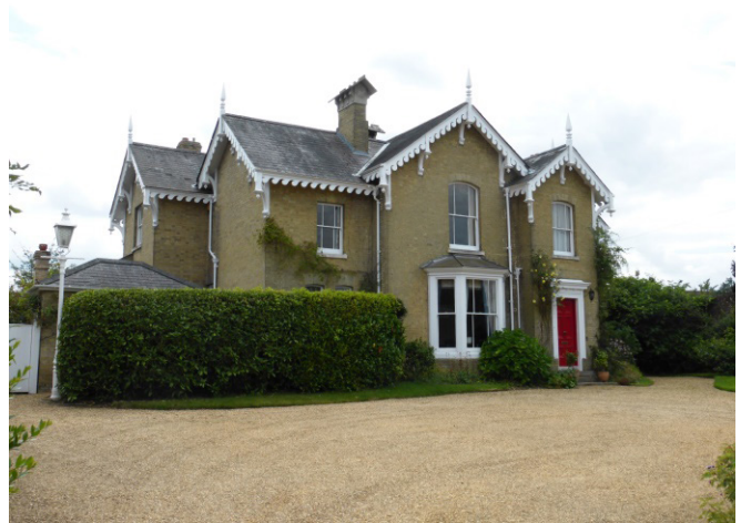
Figure 19 - No.19 High Street, Portland House
