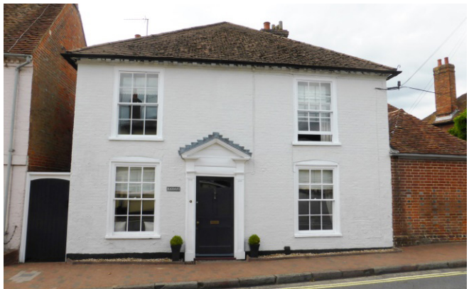
Figure 36 - No. 5 Winchester Street
