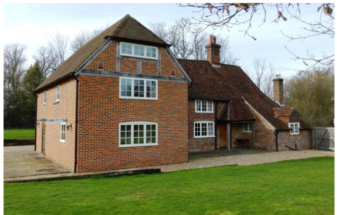
Figure 52 - Mark Farms Cottages (Farmhouse)
