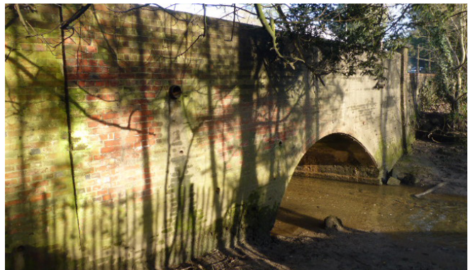
Figure 29 - Mill Bridge from downstream
