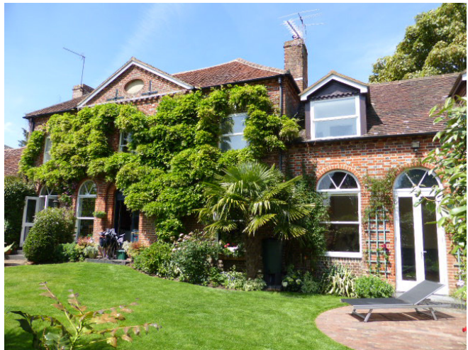
Figure 46 – Stable block to Cobbett's Cottage
