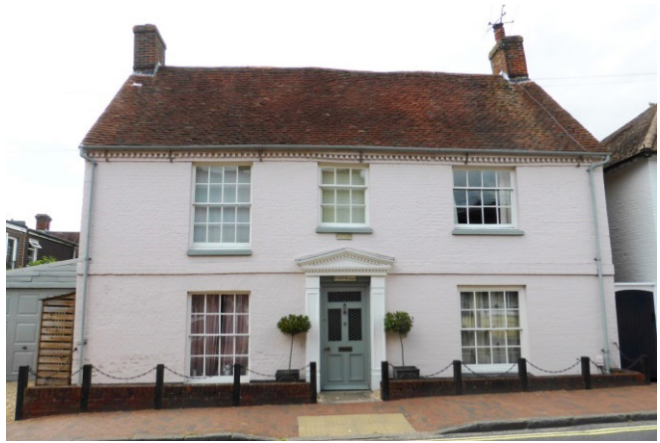
Figure 35 - No.3 Winchester Street
