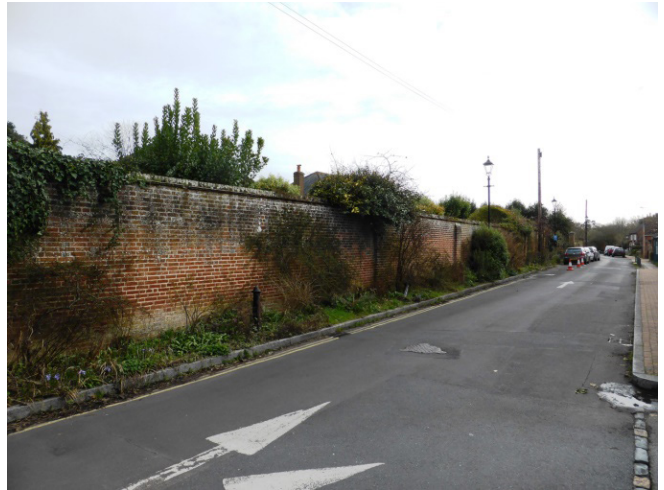
Figure 48 - listed wall on east side of Church Lane
