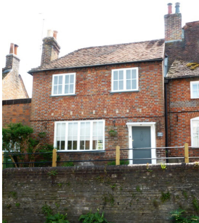
Figure 31 - No.15 Mill Hill
