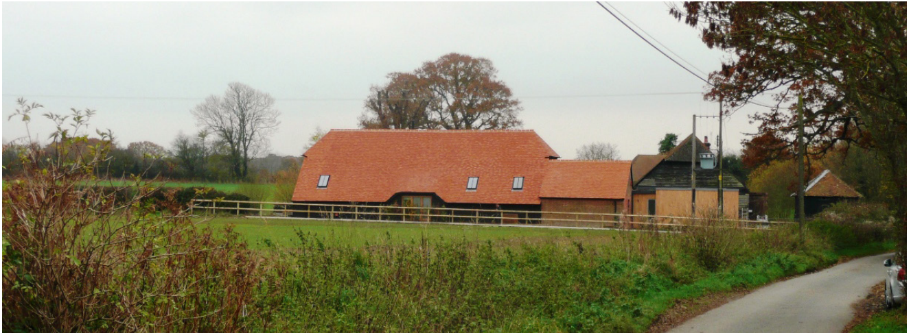
Figure 51 - General view of Marks Farm when newly roofed in 2013.
