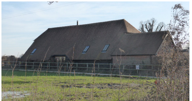
Figure 56 - Marks Farm Barn, 5 bay today
