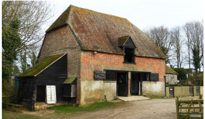
Figure 63 - Manor Farm Barn, 5 bay
