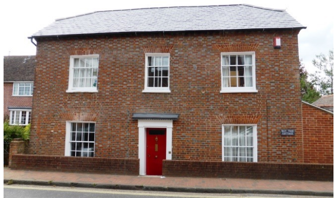
Figure 38 - No.19 Winchester Street
