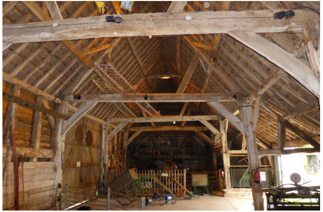
Figure 62 - Interior of 5 bay barn
