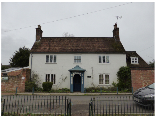
Figure 47 - No.12 (Ivy Cottage)
