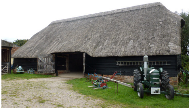
Figure 64 - Manor Farm Store/workshop
